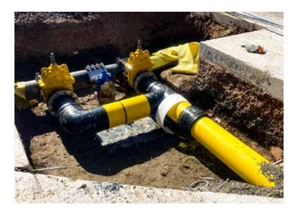
The installation project involved the deployment of a new elevated-pressure gas main, extending from the existing incoming supply housing to a newly constructed steam boiler plant room within the facility.
