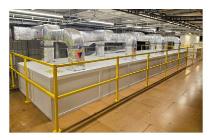
The steam tunnel area within the facility faced significant challenges due to high levels of humidity and condensation, which posed a risk to the integrity of returned clothing. A specialised climate control solution was required to maintain optimal environmental conditions and ensure that the garments remained free from moisture-related damage.
